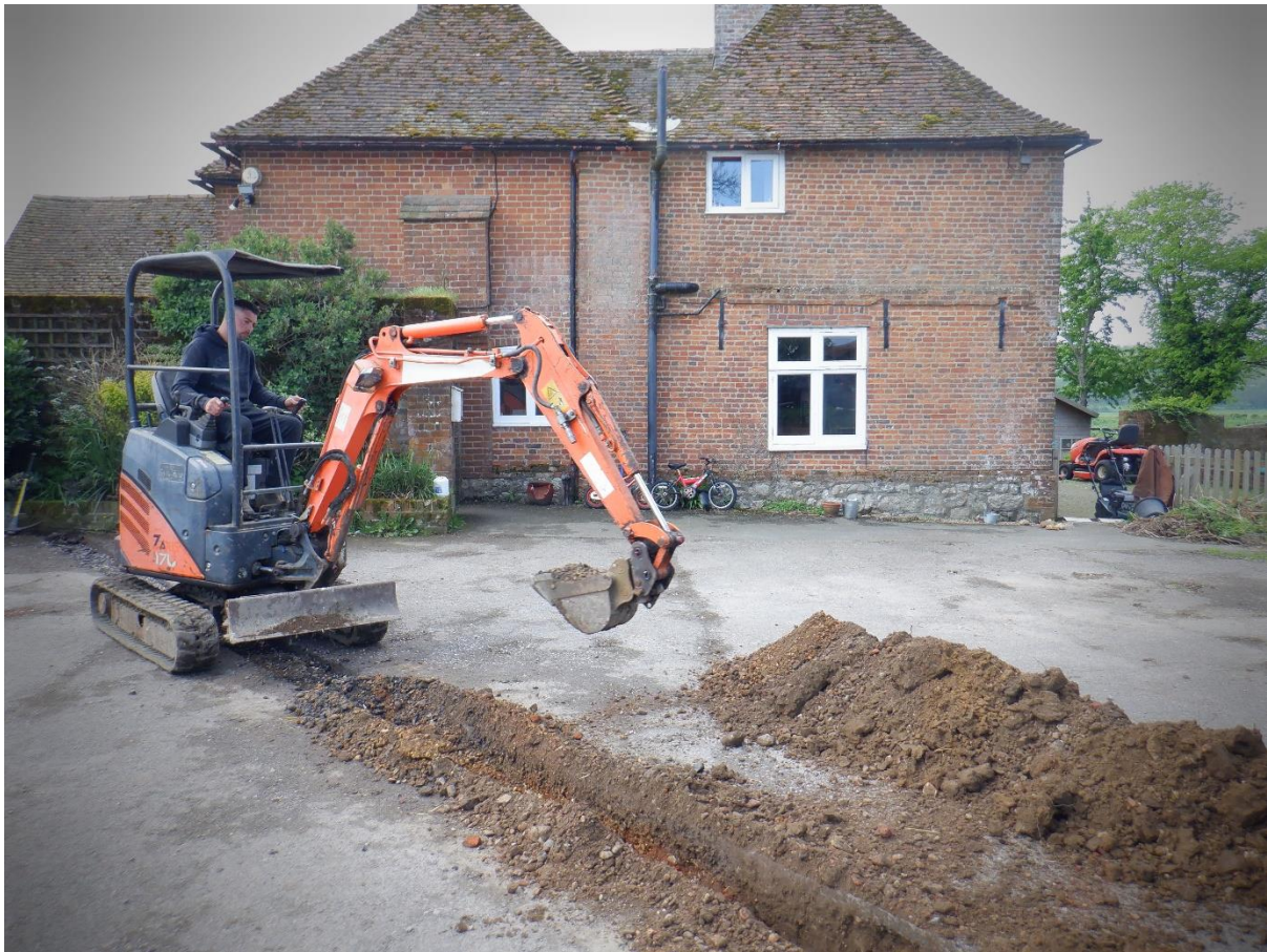
Plate 1. Setting out and starting ground reduction (looking SSW)
