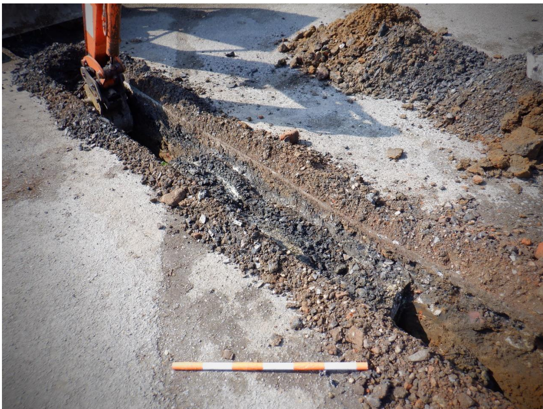
Plate 6. Modern reinforced concrete foundations (looking NNE)
