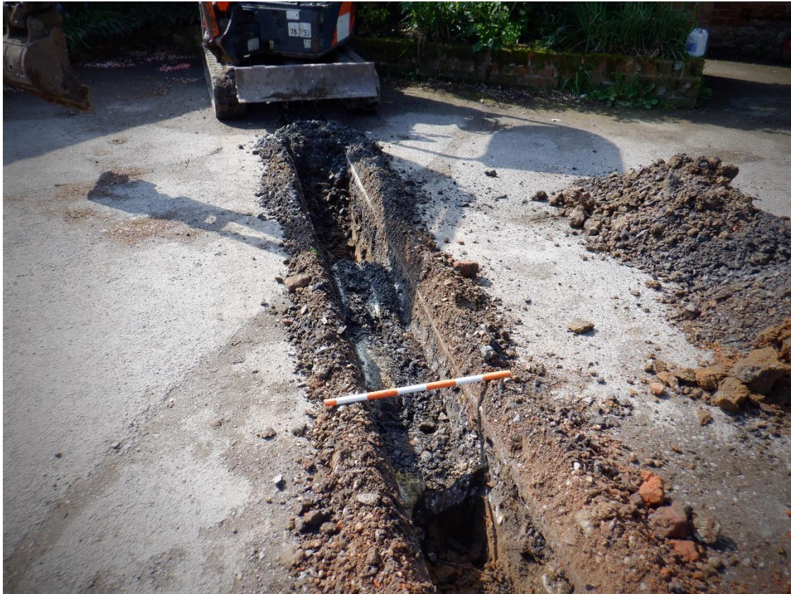
Plate 5. Exposed modern reinforced concrete foundations
